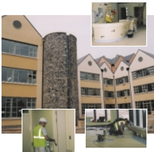
The new Naas General Hospital - good progress was made on phase 2 of the new hospital which is due to open in the last quarter of 2002
