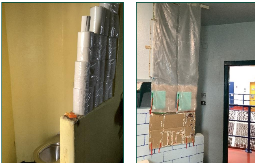
Figure 2: In-Cell Sanitary Facilities
