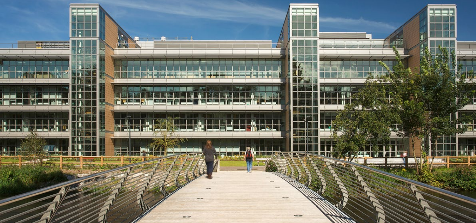
Western Gateway Building, University College Cork
