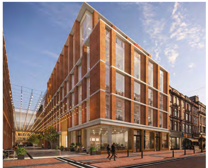
The Earl Building at Clerys Quarter - recently acquired for the Rotunda for its inner city Dublin expansion.
