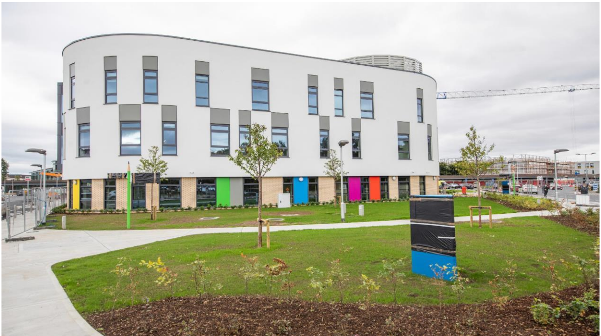
Urgent Care Centre and OPD, Tallaght Hospital, Dublin
