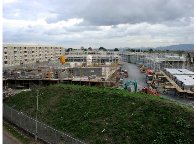
Image 3.3: New homes being built in Ballymun as part of the regeneration. Photo by John Montague.
