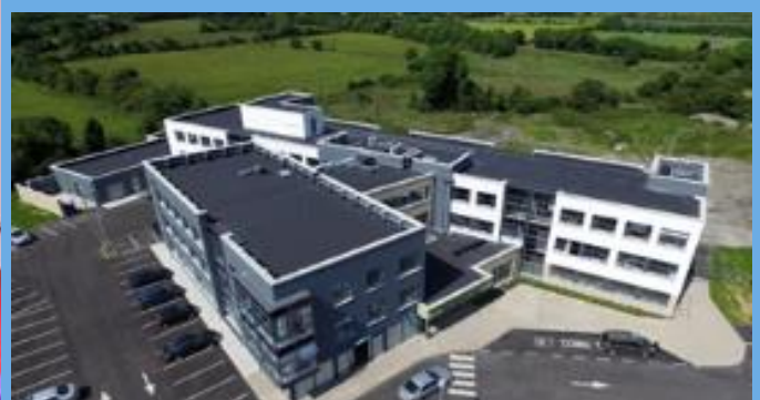
Mullingar Primary Care Centre
