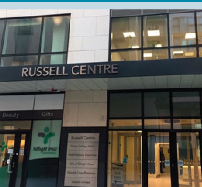
Tallaght Cross Primary Care Centre.
