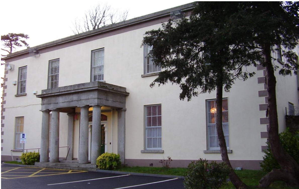
Kiltalown House Jobstown, Tallaght, Dublin 24
