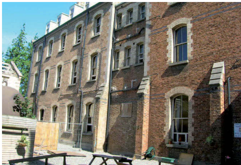
MQI High Park Residential Rehabilitation Centre, Dublin
